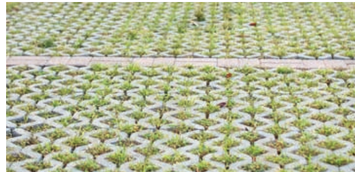
PERMEABLE PAVEMENT: A hard surface that allows rainfall to seep into underlying soils.
